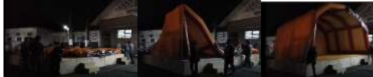
Figure 10: Installation of Inflatable Stage Roof Prototypes (6 minutes)
