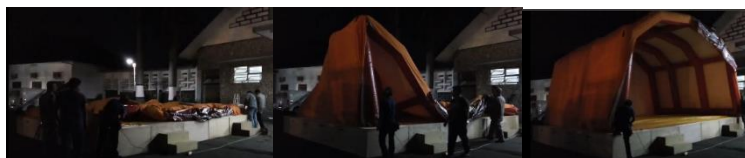
Figure 10: Installation of Inflatable Stage Roof Prototypes (6 minutes)
