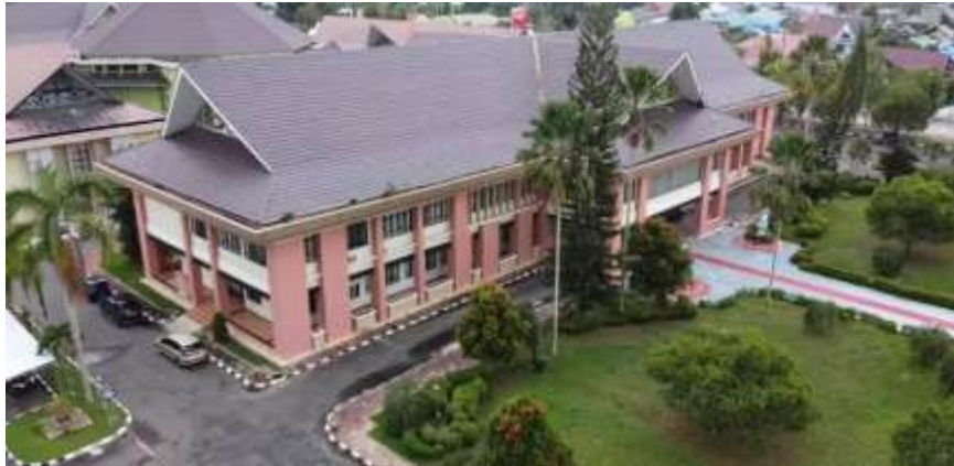
Figure 1. Kutai Kertanegara Regency DPRD Building Sumber: Kaltim. Go.id. 2020.
