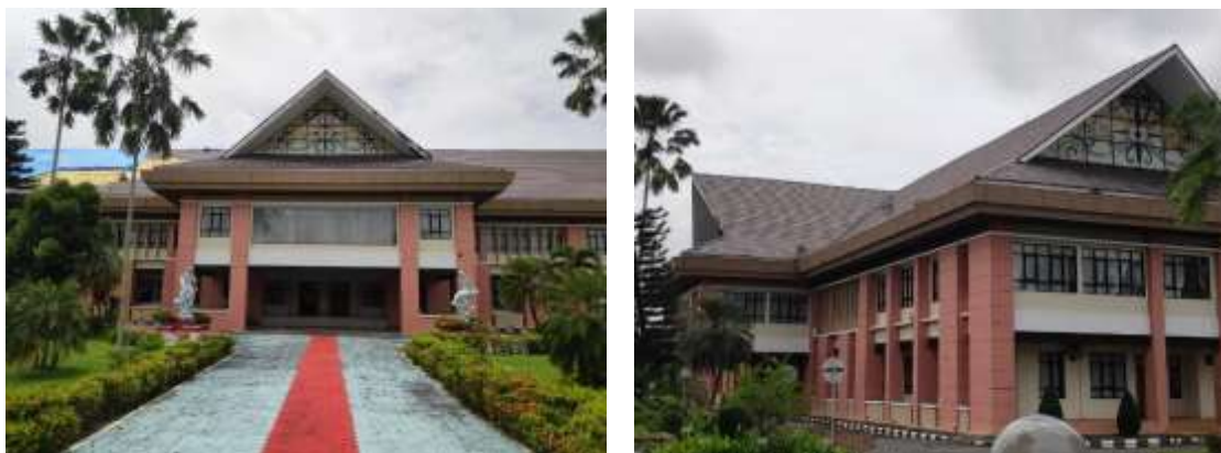
Figure 4. Kutai Kertanegara Regency DPRD Building Sumber: Kaltim. Go.id. 2020.
