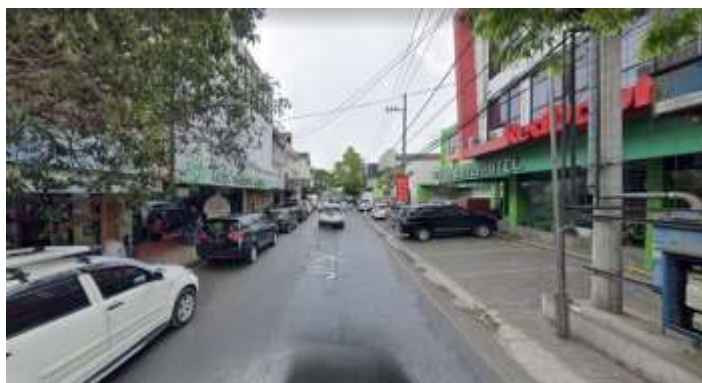
Figure 7. The Condition Of Zainul Arifin Street Malang
