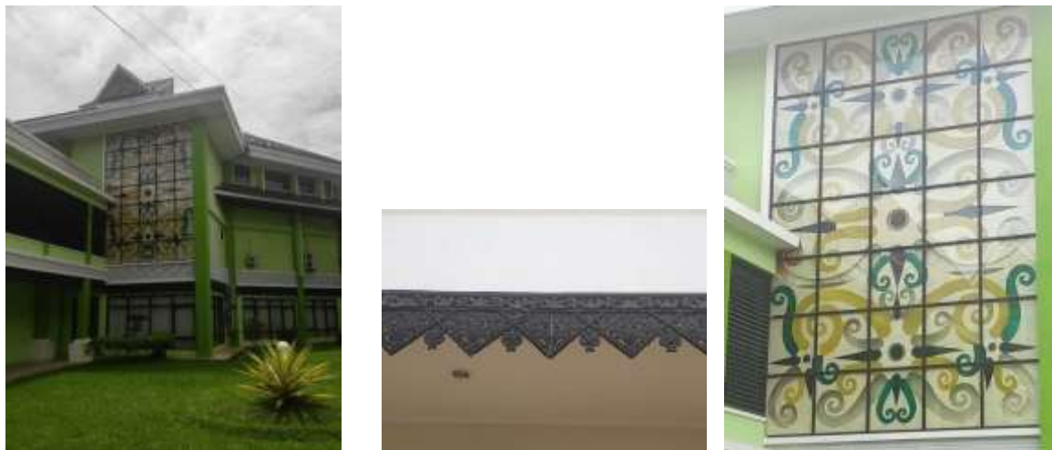
Figure 5. Kutai Kertanegara Regency DPRD Building Sumber: Kaltim. Go.id. 2020.
