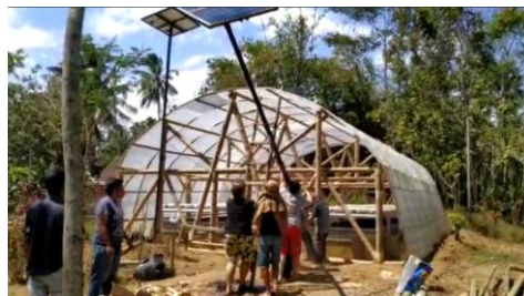
Figure 6. PLTS Installation (2 days)
