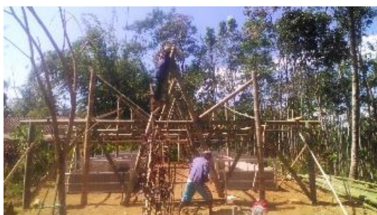
Figure 4. Construction of a Greenhouse (15 days)
