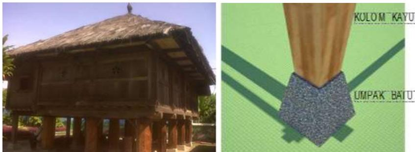
Figure 4 and 5. Kenali Traditional House and the Foundation of the Base
